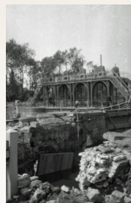
The original lock gates
