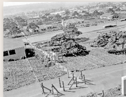
Factory camouflage - the Boeing Plant 2 in Seattle USA. The roof is camouflaged to look like a village. IWM photo
