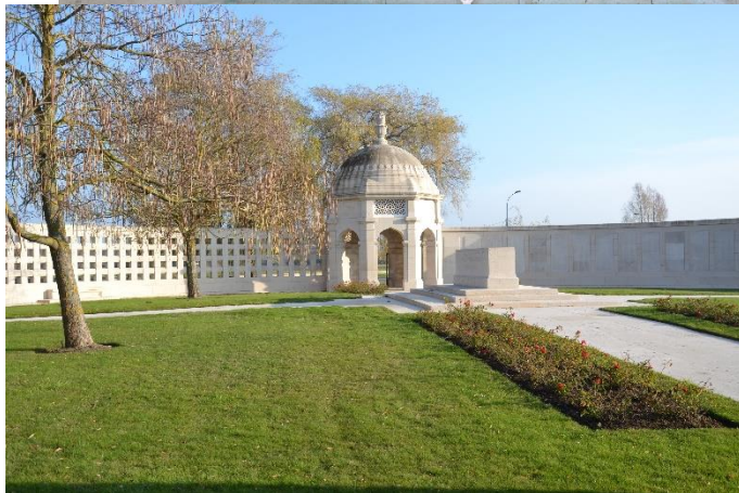
Apertured wall and dome
