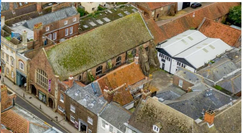
Aerial view of the St George Guildhall
